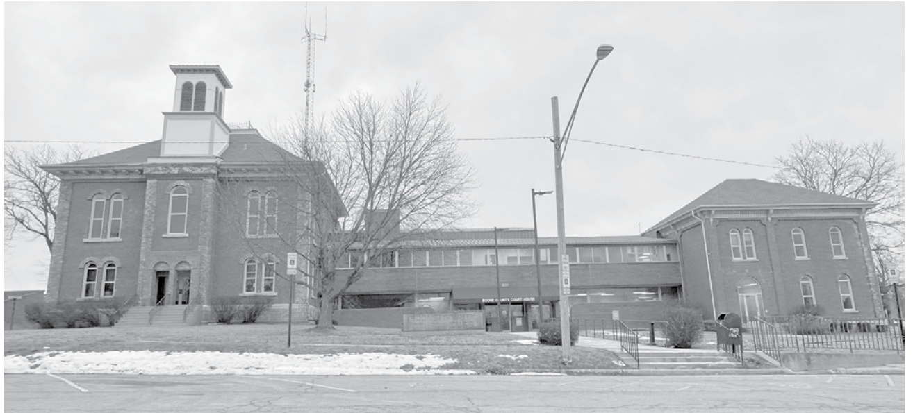
The Courthouse as it looks today, with 1970s improvements connecting the original County Clerks Building with the original Boone County Courthouse
